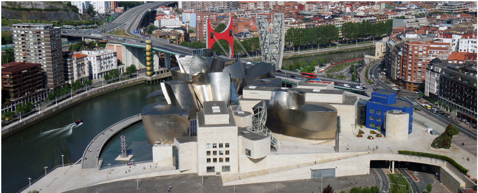
Figura 68 - Guggenheim Museum – Bilbao Espanha – Internet http://upload.wikimedia.org/wikipedia/commons/a/a1/Bilbao_05_2012_Guggenheim_Aerial_Panorama_2007.jpg
